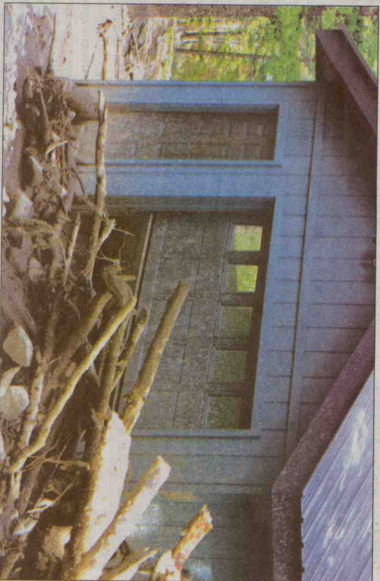
Photos by Paul J. Goetz An unidentified garage had its doors pushed in and was moved several inches on its foundation. The torrential mud and debris slide cut a new drainage channel about 30 feet wide and 4 feet deep in the foreground.
