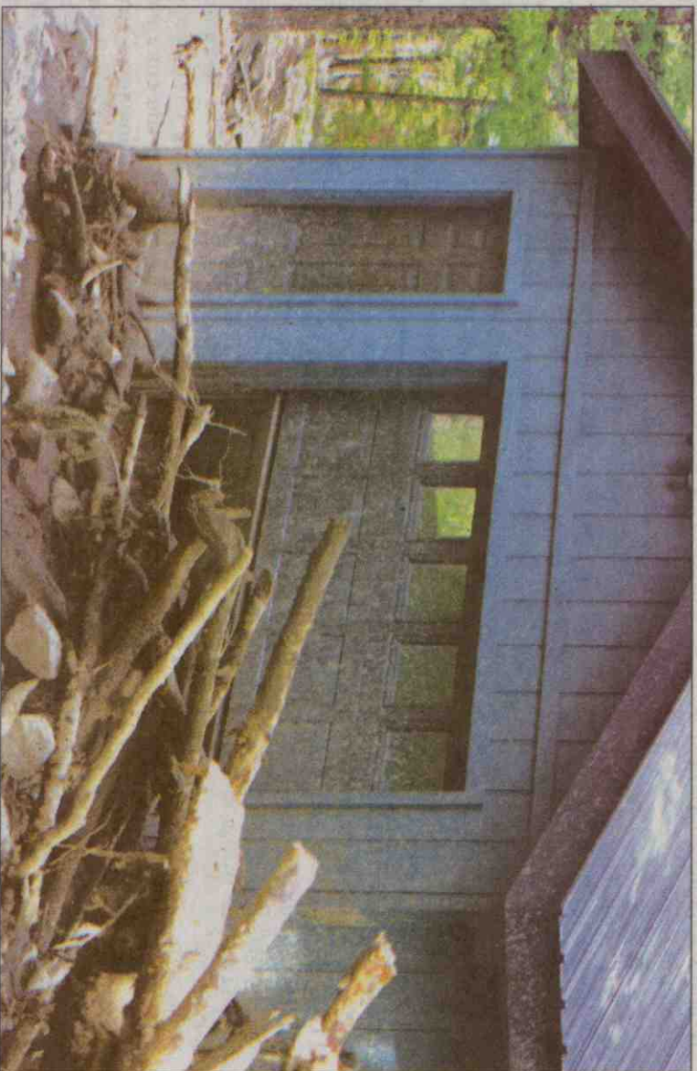
An unidentified garage had its doors pushed in and was moved several inches on its foundation. The torrential mud and debris slide cut a new drainage channel about 30 feet wide and 4 feet deep in the foreground.
